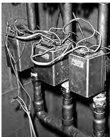
Zone valves: Separate thermostats control each zone valve. Zone valves have switches that activate the burner.
