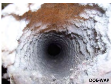
Lint collection: After years of operation, lint coats flexible pipe and eventually blocks the airway.
