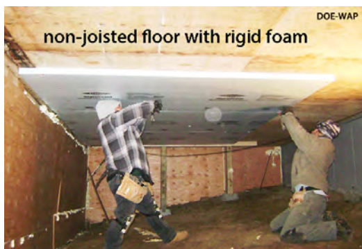
Non-joisted floors with rigid foam: Workers fasten rigid foam to a non-joisted floor with plastic-cap nails.
