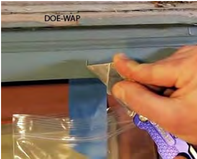
Cut through all the layers of paint. Also install a bag beneath the cut to catch paint fragments.
