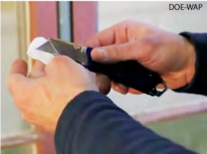
Clean utility knife to prevent contamination.
